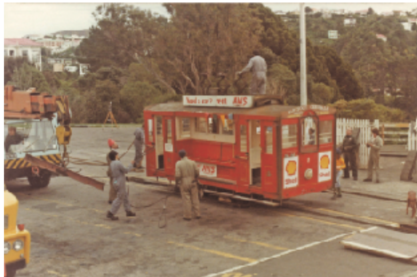
Figure 10: The construction of the Kelburn terminal
