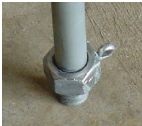
Figure 4-10: Lower Corner Spring Attachments
